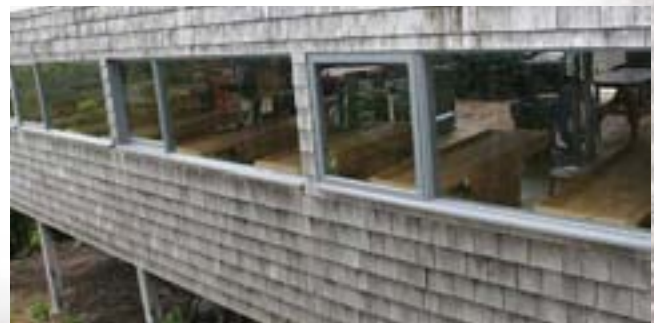
Classrooms as seen from the dining room
